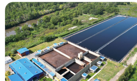
Leachate Treatment Plants
