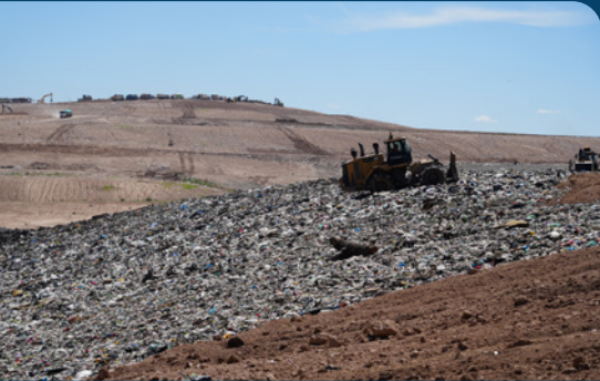
Module in the Northern Environmental Complex III
