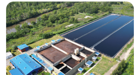
Leachate Treatment Plants
